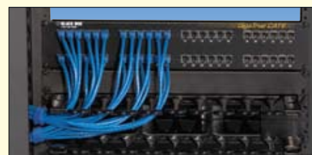
Horizontal Cable Managers keep patch cables organized.
