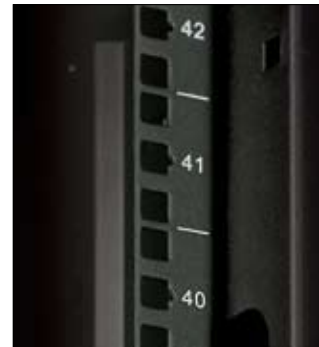
Rails are marked with rack units for easy reference.
